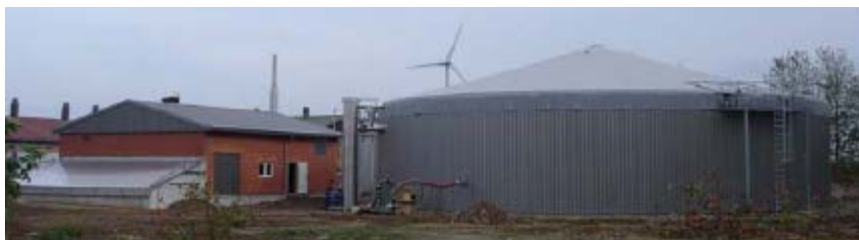
Figure 32: Biogas and wind power plant in Feldheim
